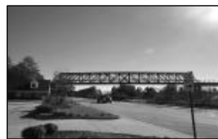
Golf Cart Bridge crossing GA Hwy 74
